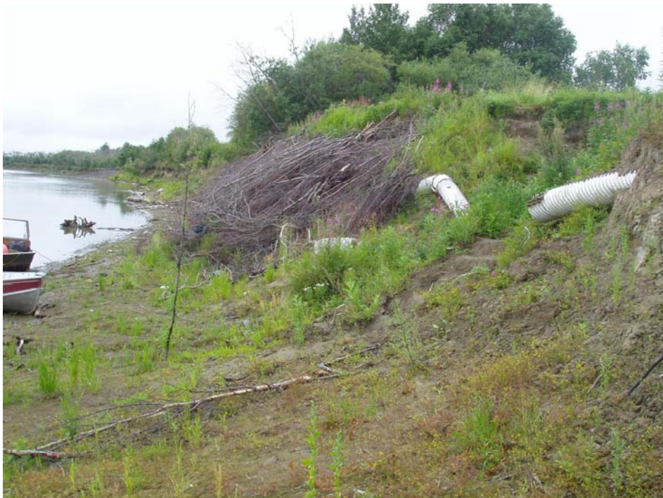
N 61° 32.267' W 160° 19.120' Upper Kalskag P1011167 Photo 2. Looking downstream, 4" arctic pipe exposed.
